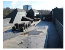
Wall mounted overflow scuppers should also be checked for water tightness and possible internal leakage, particularly on discharge shingle side.
