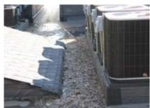
4. It is recommended that an in-house roof maintenance program be established to clean the rubber roof on a quarterly basis of leaves and other debris, to minimize clogging of the roof drains and overflow scuppers.
