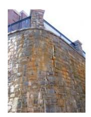
6. Repair all cracks located on the east face of the front retaining wall. Have all repairs reviewed and approved by a licensed structural engineer prior to and after completion.
