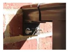
3. Properly seal the large open joint under the metal sill plate on the exterior balcony of unit 402.
