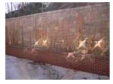
4. Power wash the efflorescence and red clay staining from the stone retaining wall at the south of the This will have to be building. redone periodically.
