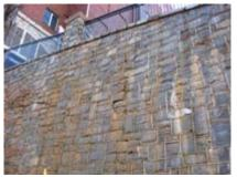
7. Repair the large crack in the front retaining wall approximately half way along the length of the wall. Have all repairs reviewed and approved by a licensed structural engineer prior to and after completion.
