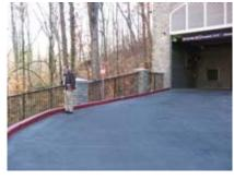
7. There is a large drop off on each side of the entry bridge. Investigate adding bollards, or an automotive guardrail, on each side of the entry.
