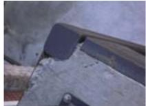
2. The wall attachment bolts utilized on the anodized aluminum balcony railings on the east elevation appear undersized. Confirm code adequacy of the attachment bolts at all locations.
